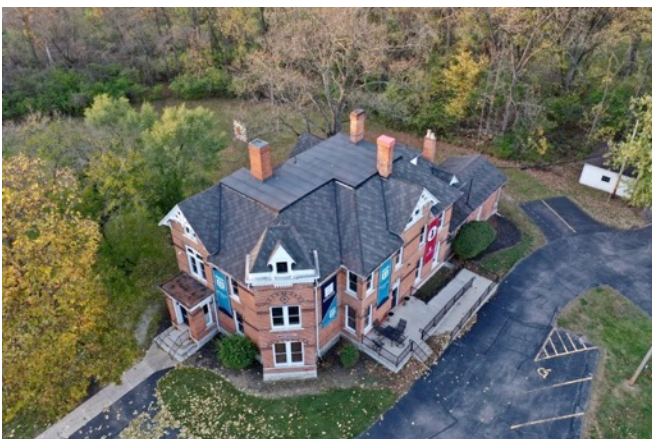
Browne Hall and Parking Lot
