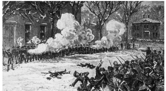
Springfield Armory, January 25, 1787. In reality the two sides were over 100 yards apart, and it was artillery fire that scattered the Regulators
